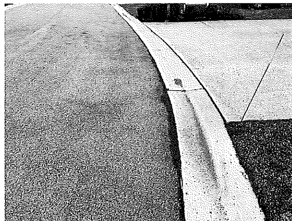
Concrete gutter
