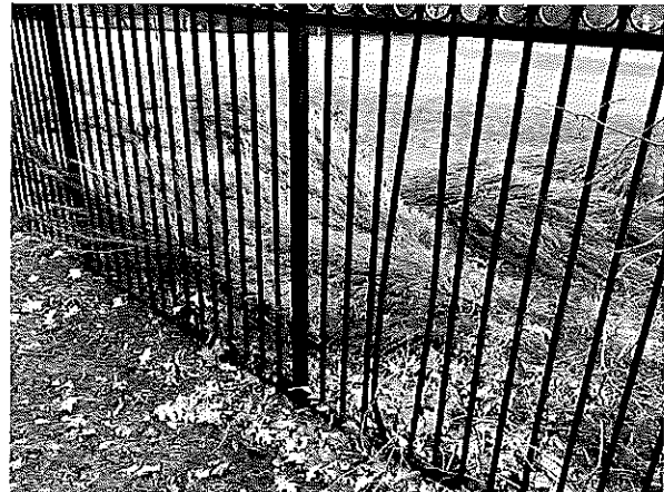
Fence picket damage
