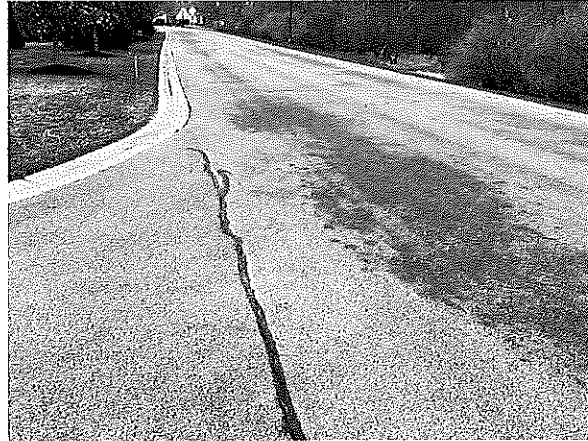
Crack repair
